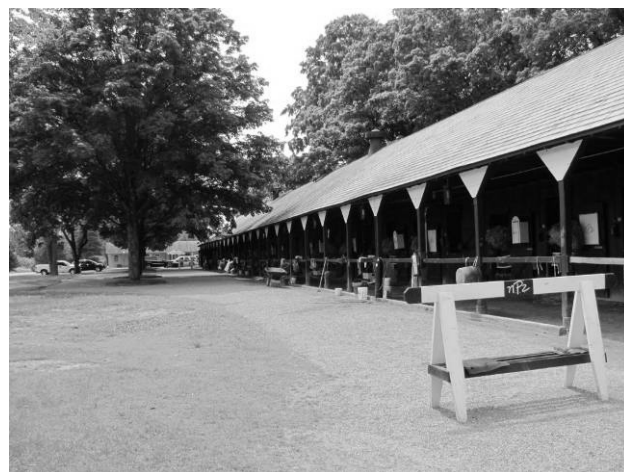
The environs of barn #84, occupied by Nicholas P. Zito's establishment, has been enhanced by the addition of peastone paving, wood timber trim around the bases of trees, and tables, chairs and umbrellas for outdoor eating.
