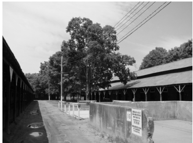
A muck storage bin at Madden Court typifies the crude, unfinished look of this ubiquitous Backstretch feature.
