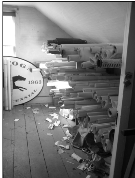
View of "plan room" on the second floor of Building #68. While a hand written list of these rolled architectural drawings does exist, there is no searchable database or any method in place for protecting these important archival resources.
