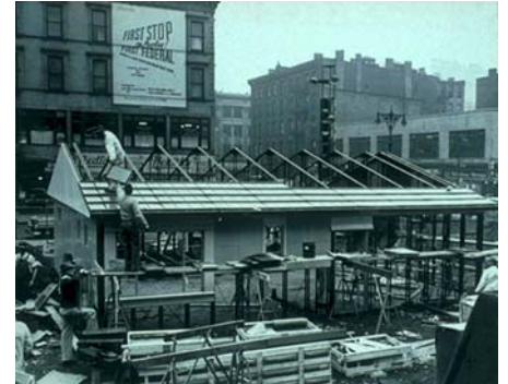
Fig. #2 - Construction of first model house in New York City.
